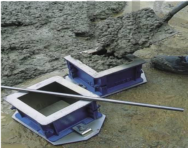
Fig. 2. Casting of Concrete Cubes (M50)
